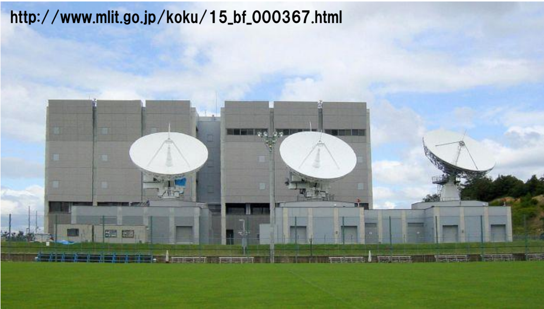
QZSS Control Center Kobe,
