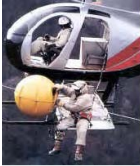
Figure A-14. Aerial marker being attached to a power line from a helicopter
